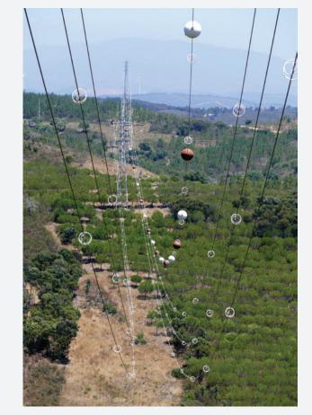
involves projecting ultraviolet light Multiple bird flight diverters installed on a transmission line. Algarve region, Portugal. Photo: Alvaro Camiña along power lines to increase visibility
